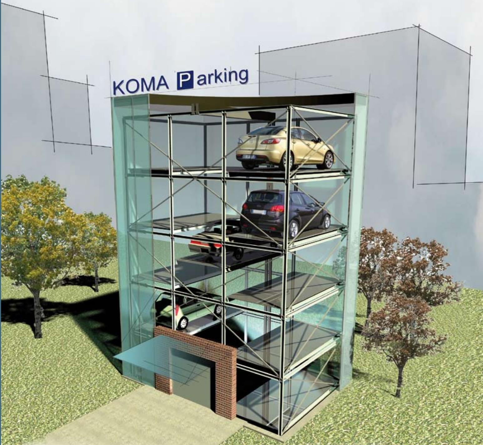
An automatic system for independent parking, based on stacking cars and shifting pallets to either side of the lifting device. As required, several installations can be placed side by side or linked one after another.
